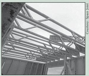
Trim-able Floor Trusses are a hybrid of truss and I-joist technology.
