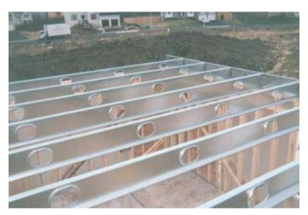
Pre-Punched Steel Floor Joists Image Source: PATH (www.pathnet.org)
