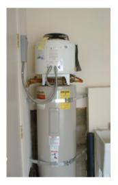
E-Tech R-106 mounted on a storage tank Image Source: <u>www.aeretech.com</u>
