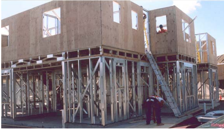
Figure 1 - Hybrid steel-wood home at Radford Terrace.
