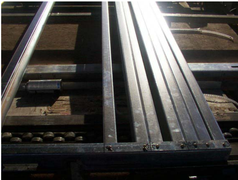
Figure 2 – Multiple members built off-line and placed on main panel table.
