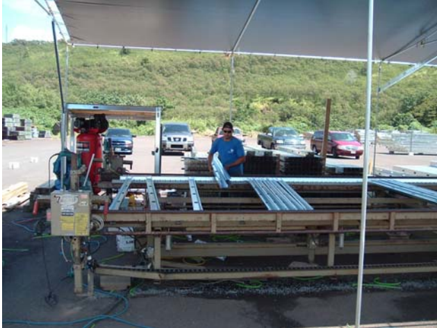
Figure 3 – Framing table at plant
