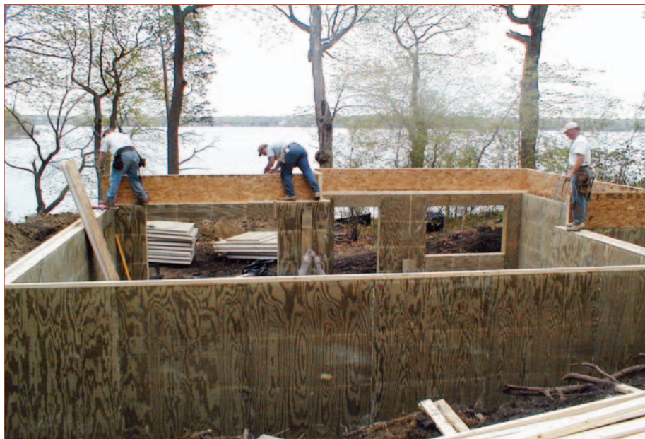
With below-grade SIPs, a 5-ply, 2x4 treated glulam functions as the stud, supporting the dirt load against the outside.
