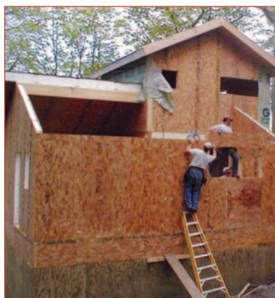
The installation had to be done in stages because there wasn't a second floor in part of the house. Also, the crew had to leave the back wall until last to provide an entrance for the upper wall panels.
