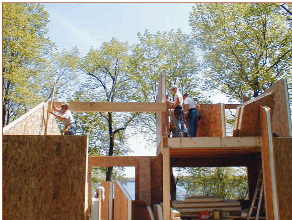
Once they got the floors in, Stendel's crew could add the upper wall panels and the SIPs roof system.
