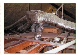
HVAC and ducts are located in conditioned space because of insulation in the roof line. The unit was also strategically placed in the middle of the attic to shorten duct runs.
