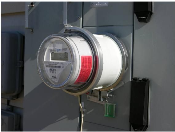
Figure 3 – Enetics Equipment Installed between Utility Meter and Meter Housing
