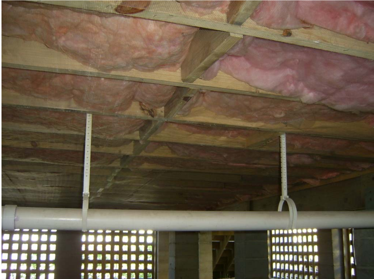
Figure 1 – Typical raised floor foundation
