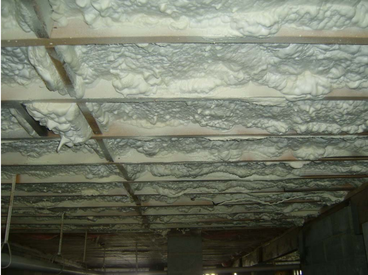
Figure 4 – Icynene insulation between joists of raised floor system.
