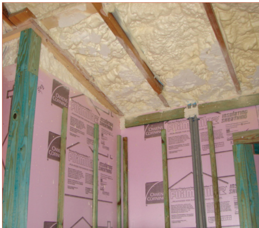
Black blew Icynene under the roof decking and along the top portion of the walls adjacent to the cathedral ceilings.
