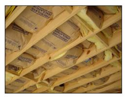
Photo of improperly installed insulation. Insulation loses effectiveness when compacted (EnergySense photo)
