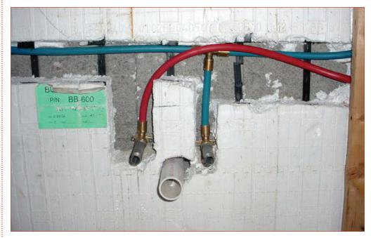
With PEX piping, small-diameter tubing can be used in parallel installations-like this one for a sink-to limit water consumption while waiting for delivery of the heated water. There is also less heat loss from PEX pipe than from metal pipe.
