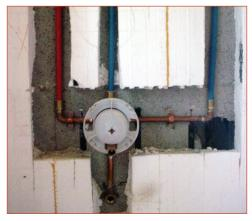
PEX piping, which ranges in size from 1/4 to 2 inches, is lightweight and flexible, allowing Brothers Strong to easily work the hot and cold supply lines through insulation to reach a shower valve like this one.
