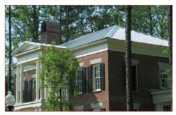
Following the architect's recommendation, Hastings used a standing seam metal roof, which offers greater efficiency and durability—and less maintenance—than a traditional roof.
