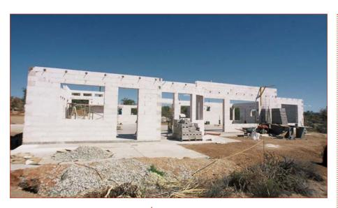
Walls built with AAC block are consistently straight, but can also be sculpted to meet a variety of architectural designs.
