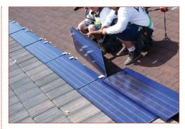
Carefully interconnecting each module, two crew members tie in the first two rows of the integrated PV system with the concrete roofing tiles.
