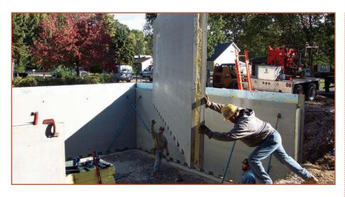
Workers maneuver a precast concrete wall panel before it is braced and welded in place.
