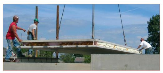
The erection crew positions a precast concrete floor panel with assistance from a crane.
