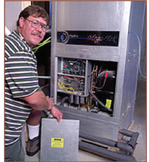
A homeowner in Colorado shows off his geothermal heat pump. Photo courtesy of the U.S. Department of Energy's Office of Energy Efficiency and Renewable Energy.
