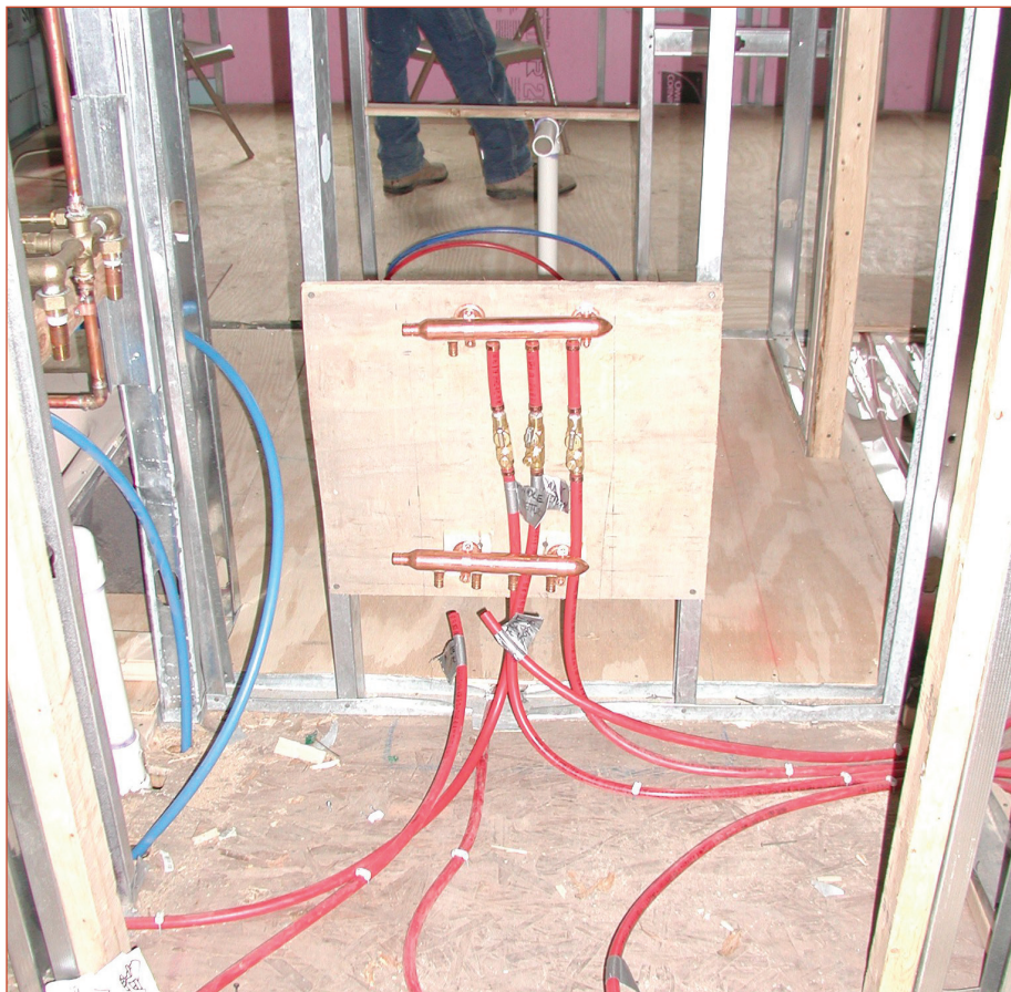
This radiant heating system uses PEX piping to transport water for heating.
