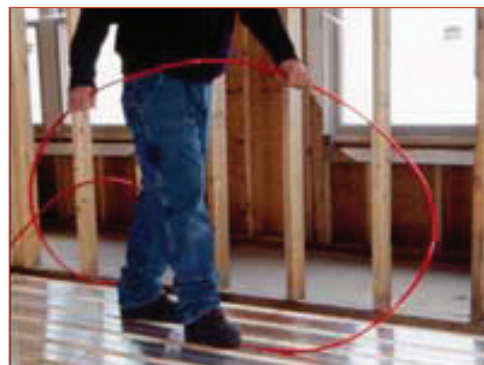
PEX piping is easily uncoiled and quickly embedded in the floor.
