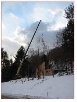
Vermont Built uses a six-man crew with a minimum of two men on the deck, one man on the truck hitching the chain, and one operating the crane. This allows the crew to set the walls for the first and second floors in two days.
