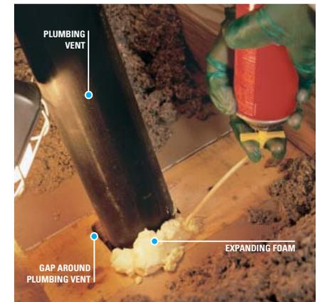
If the space around your plumbing pipe is wider than 3 inches, you may need to stuff some fiberglass insulation into the space to serve as a backer for the expanding foam. Once the fiberglass insulation is in place, follow the directions on the can to foam the space around the pipe.
