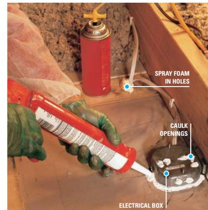
Fill wiring and plumbing holes with expanding foam. Caulk around electrical junction boxes, and fill holes in box with caulk.
