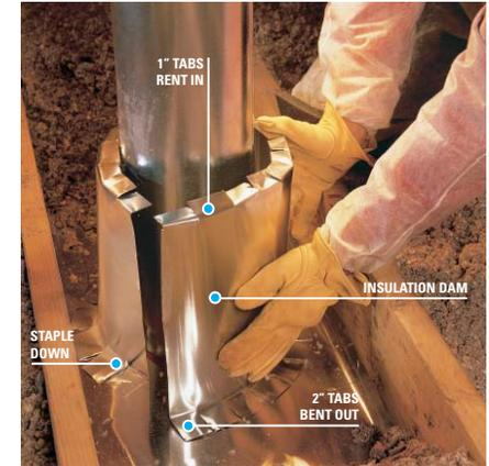
Form an insulation dam to prevent insulation from contacting the flue pipe. Cut enough aluminum from the coil to wrap around the flue plus 6 inches. Cut slots 1 inch deep and a few inches apart along the top and bend the tabs in. Cut slots about 2 inches deep along the bottom and bend out the tabs. Wrap the dam around the flue and secure the bottom by stapling through the tabs. Now put insulation back right up against the dam.
