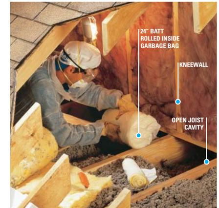
Cut a 24 inch long piece from a batt of fiberglass insulation and place it at the bottom of a 13-gallon plastic garbage bag. Fold the bag over and stuff it into the open joist spaces under the wall (a piece of rigid foam board sealed with spray foam also works well for covering open joist cavities). Again, cover with insulation when you're done.
