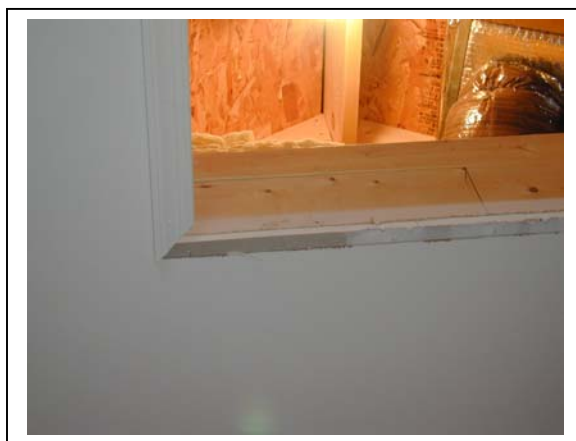
Figure 13 Attic Hatch Opening
