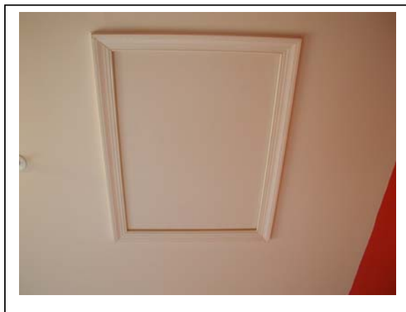
Figure 16 Finished Hatch in Place
