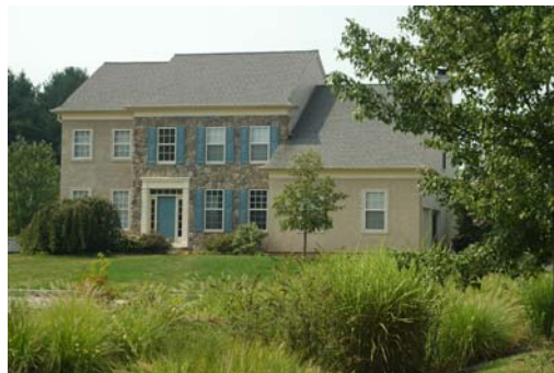
Figure 3. Field Investigation. Single-family Residence in Ambler, PA
