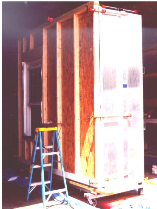
Figure 6 Wall Secured in Test Chamber
