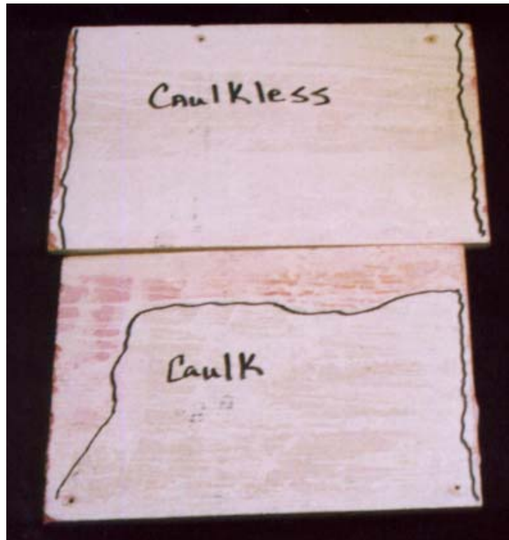
Figure 12 Fiber Cement - Staining on Back of Siding (Extent of Staining is Outlined)
