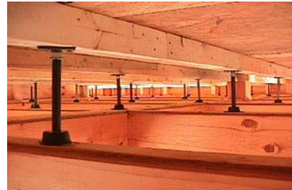
Raised Floor Above Joists
