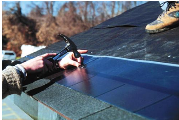
PV Roof Shingle Installation Image Source: www.toolbase.org
