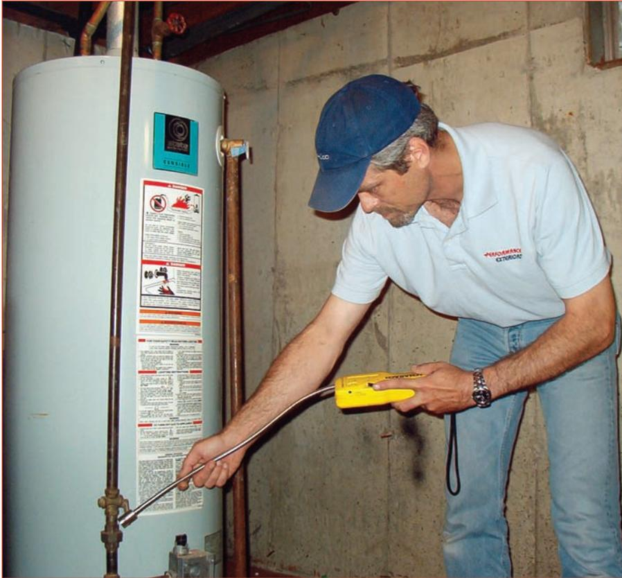
Lotesto tests the water heater gas lines for leaks.
