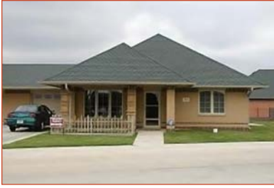
In his bid to build the model home, David Ritchie included plans for an energy efficiency package, including geothermal heat pumps.
