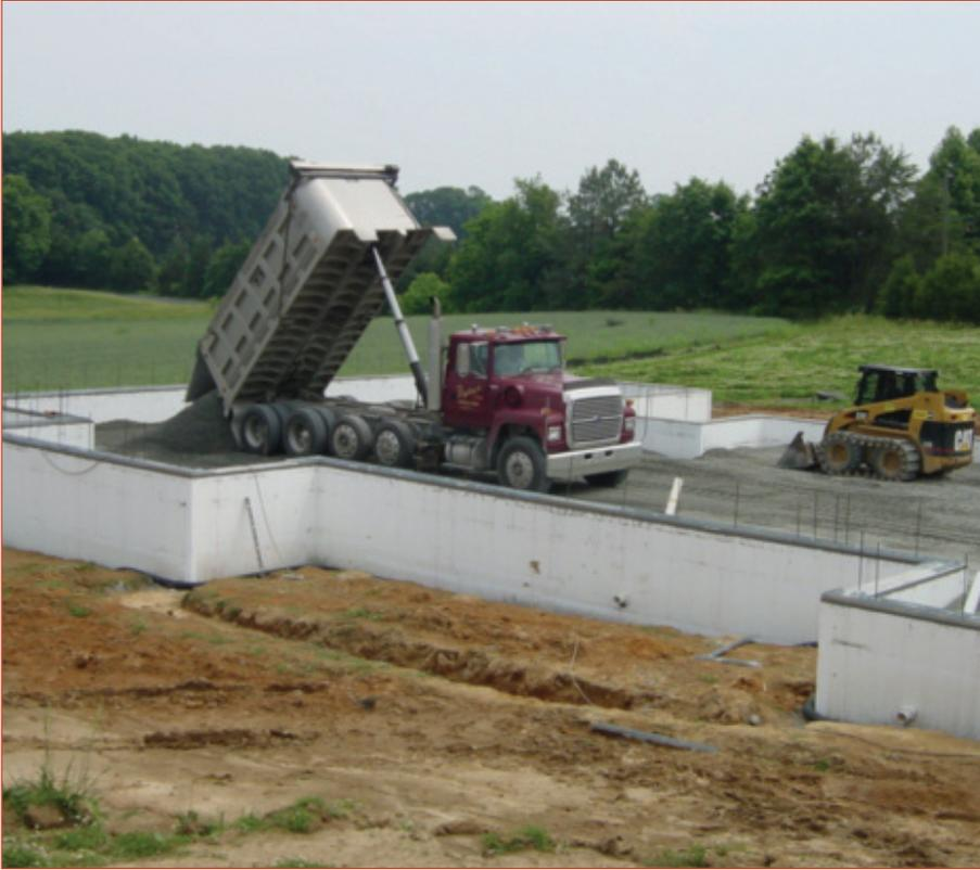
Vertical ICFs are strong enough to withstand many tons of weight without backfill.
