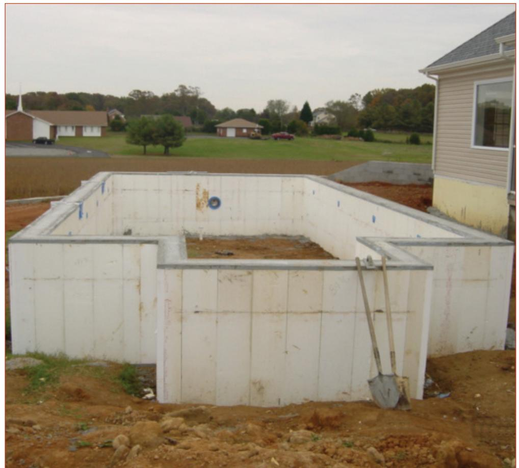
Arrington used excess vertical ICFs to construct a 16' x 32' in-ground pool.
