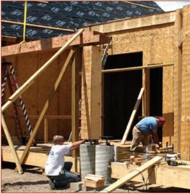
With synthetic roof underlayment, the Hearthstone crew has a reliable six-month temporary roof that allows them to work through different seasons.
