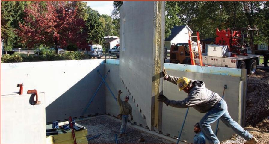
Workers maneuver a precast concrete wall panel before it is braced and welded in place.
