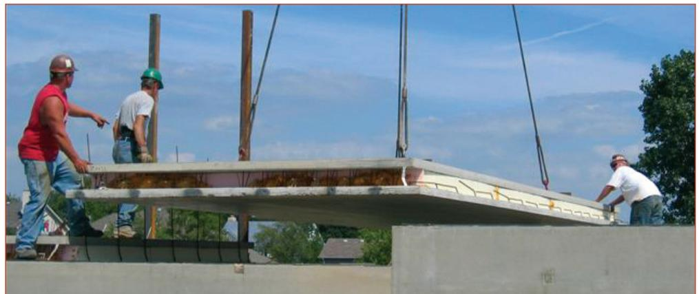
The erection crew positions a precast concrete floor panel with assistance from a crane.
