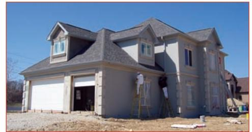
Built with precast panels, this home is designed to withstand natural disasters, including an F-4 rated tornado.
