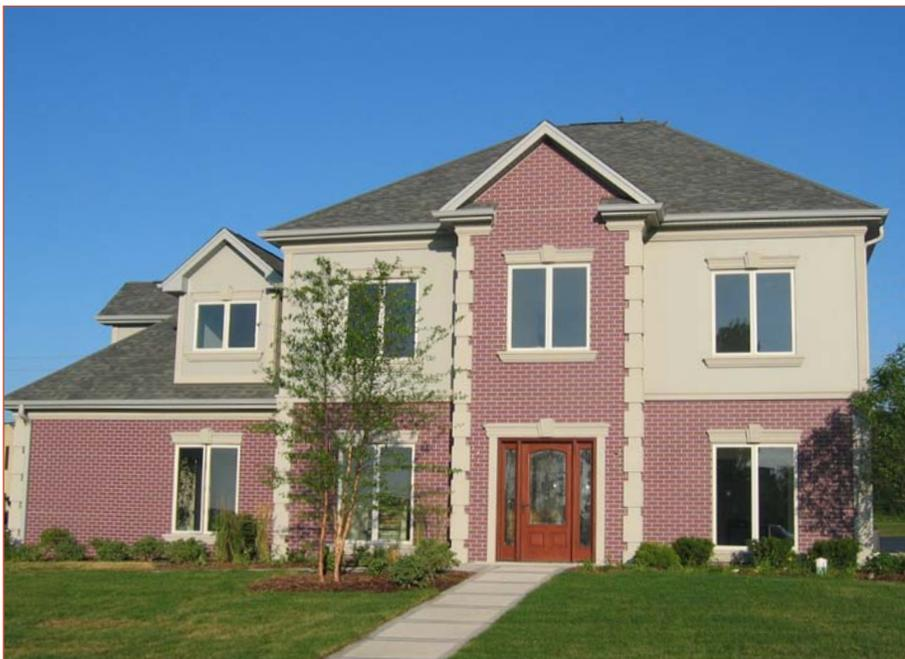
Concrete form liners are used to create exterior finishes ranging from brick to stone, which are painted in the field.
