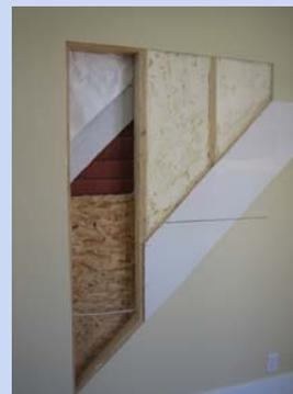
Advancements in building envelope construction can be seen through the "truth window" in the great room, which provides a cut away through the dry-wall, insulation, wood framing, weather barrier, and siding insulation, and ends at the Autumn Red siding.
