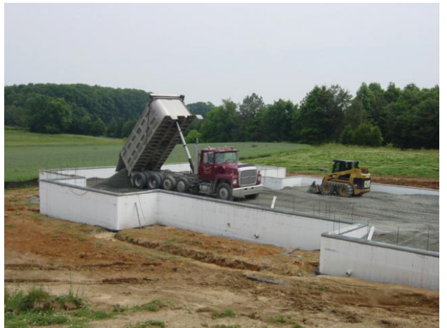
Vertical ICFs are strong enough to withstand several tons of weight without backfill.
