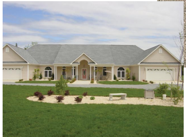
Arrington has completed five projects using vertical ICFs. The first home she built was for herself, she says, and she followed the manufacturer's manual to help her along her way.
