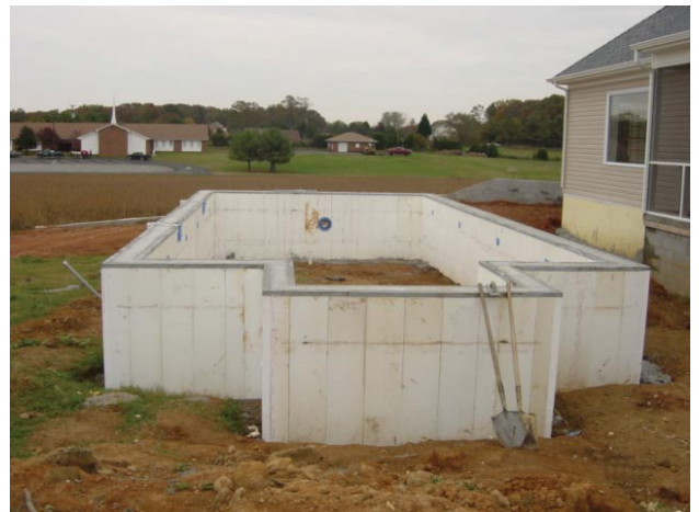
Arrington used excess vertical ICFs to construct a 16-by-32-foot in-ground pool.
